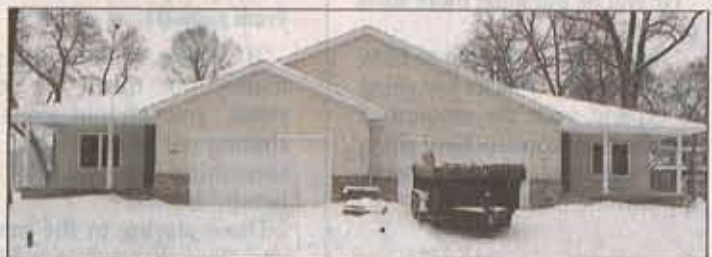
Bruce Newton is renovating, redeveloping and building homes on available lots in the Cedar Heights Elementary School neighborhood. One of Newton's nearly-finished products, on Hawthorne Drive in Cedar Falls, is shown at left.
